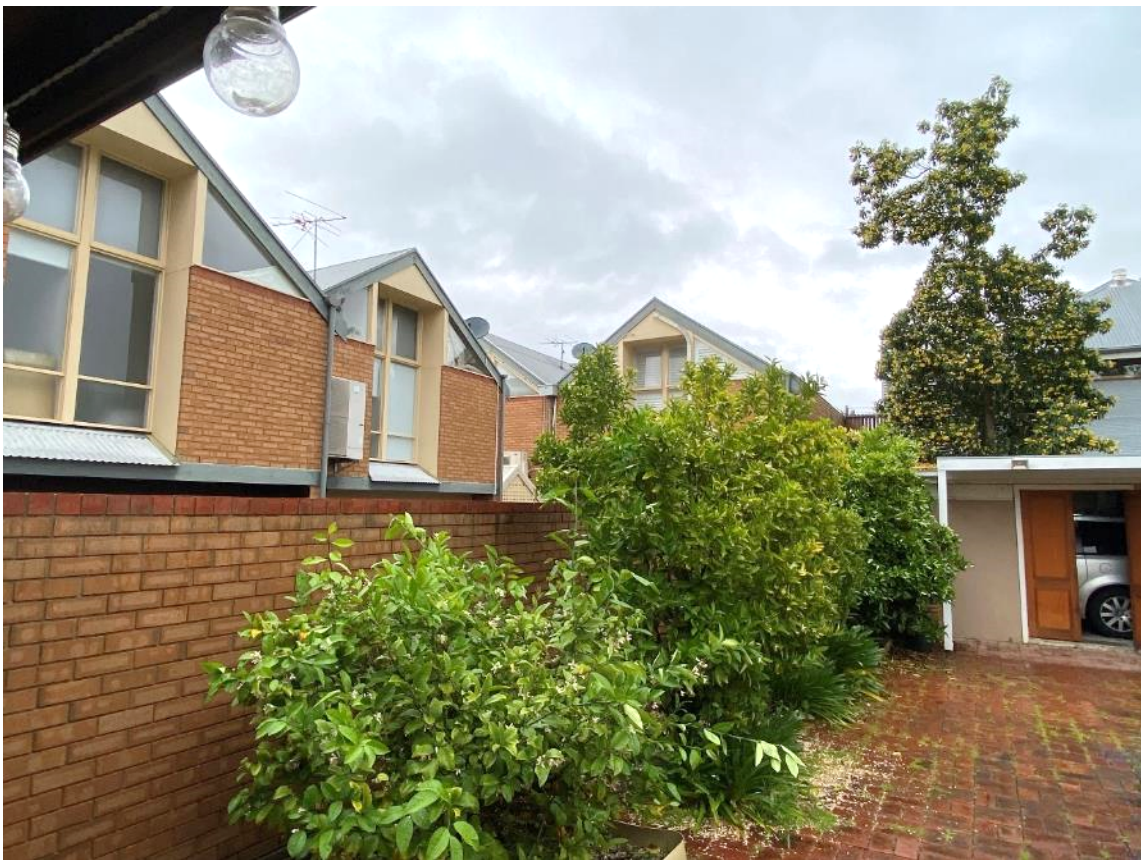
Photo 3.4 – private open space and southern boundary wall
