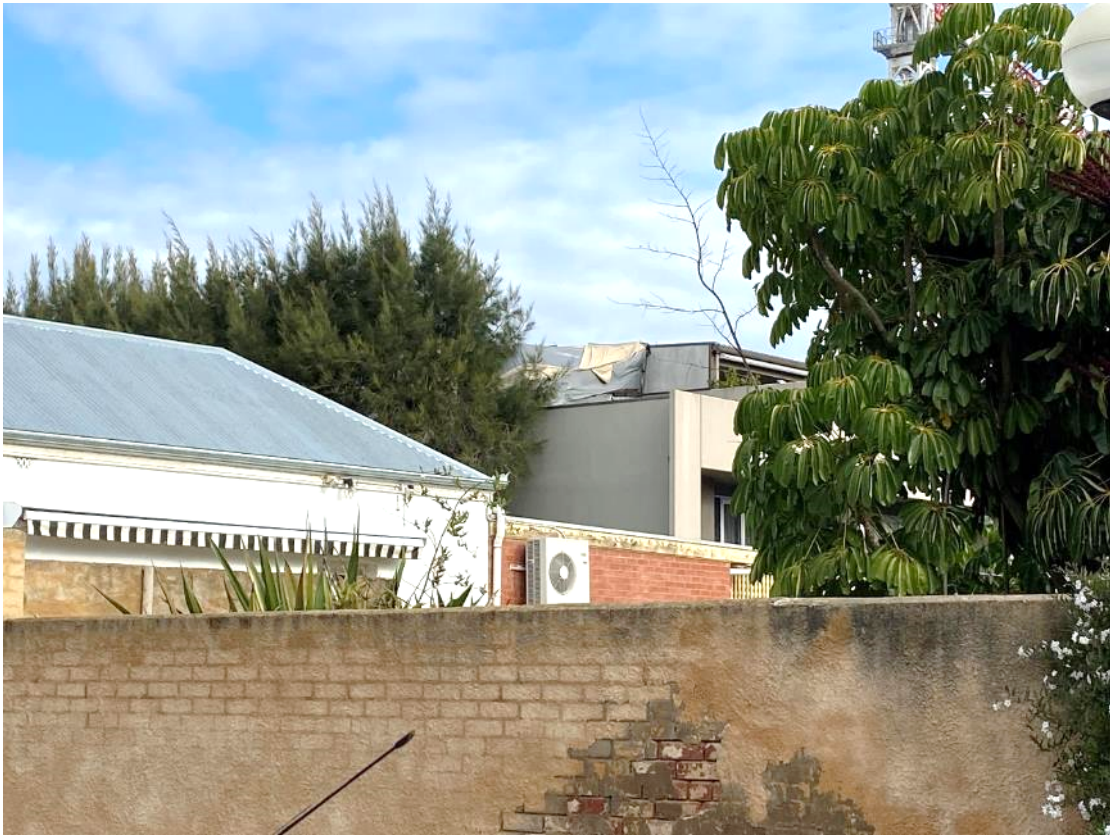
Photo 3.5 – subject site rooftop visible from Curtis Street
