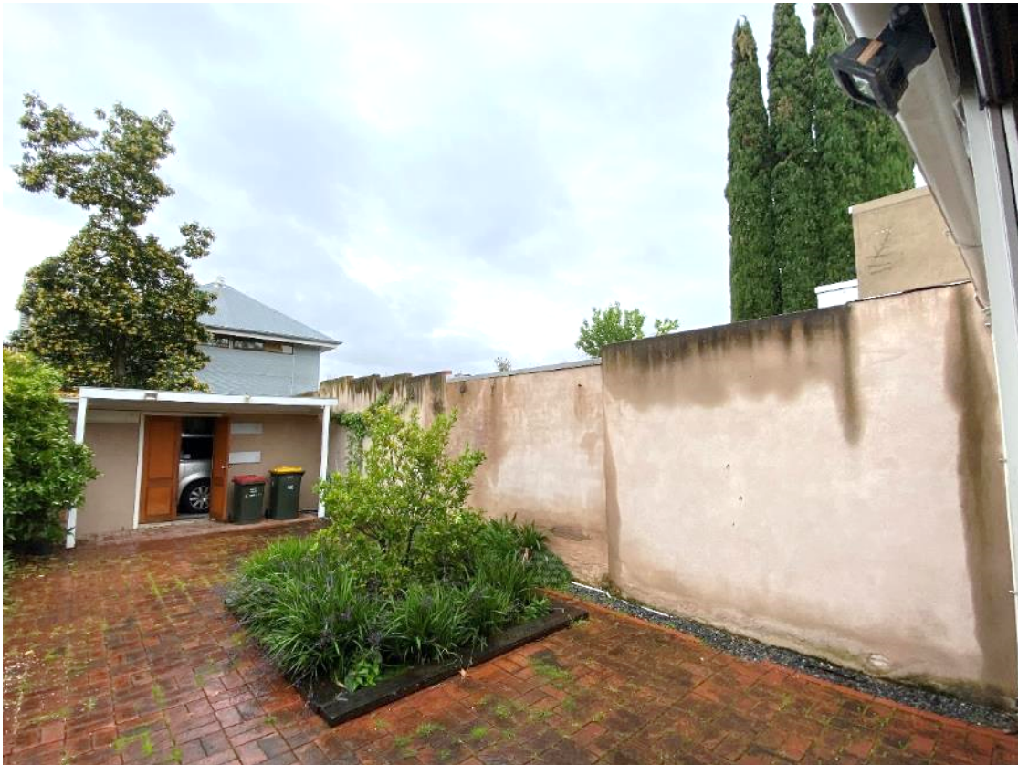
Photo 3.5 – private open space and northern boundary wall
